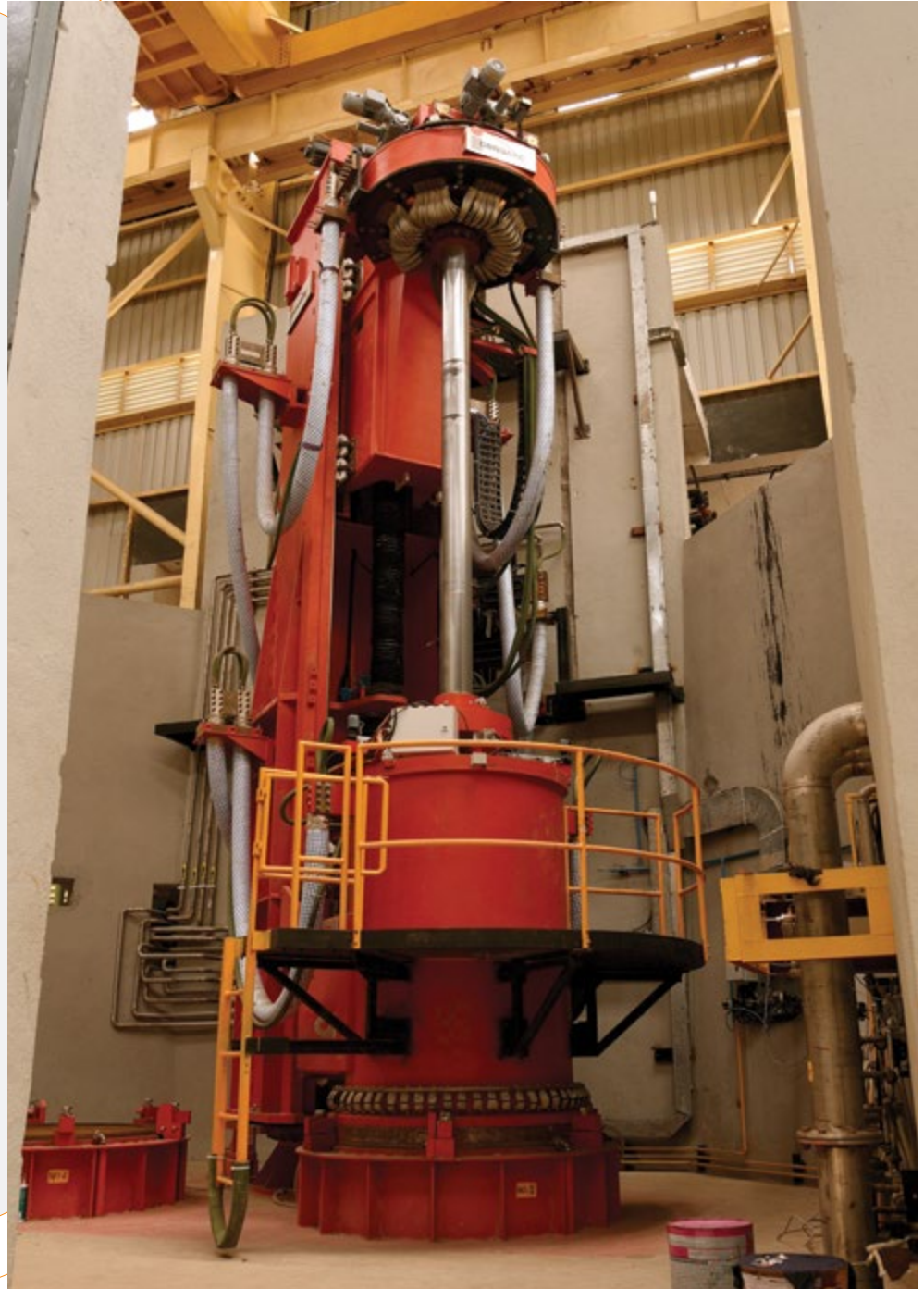
▲ 10T Capacity Vacuum Arc Re-melting Furnace at new Titanium Plant
